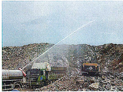
矿山作业洒水车抑尘
